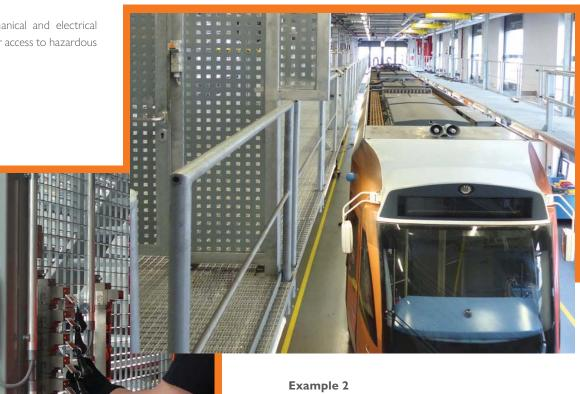
After the overhead lines have been isolated, a key is removed and the working platforms can then be accessed. Maintenance personnel must then remove a protection key to unlock the access door. The doors can also be equipped with escape releases so that everyone can leave the danger zone if a door is closed behind them and then leave the hazardous area as quickly as possible in case of danger.
